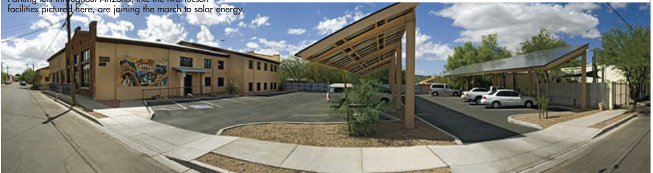
Parking lots throughout Arizona, like the two Tucson facilities pictured here, are joining the march to solar energy.
